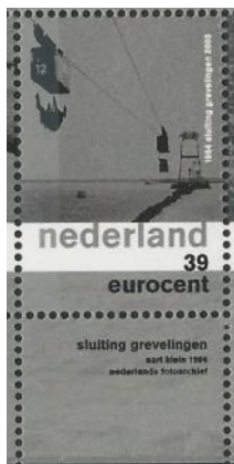
Figure 19: Cable cars were used to close the Grevelingen dam.
