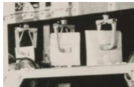
Figure 10b: This detail of the center of Figure 10a illustrates the gripping and rotating mechanism by which the letters were fed in the correct position along a stamp head.
